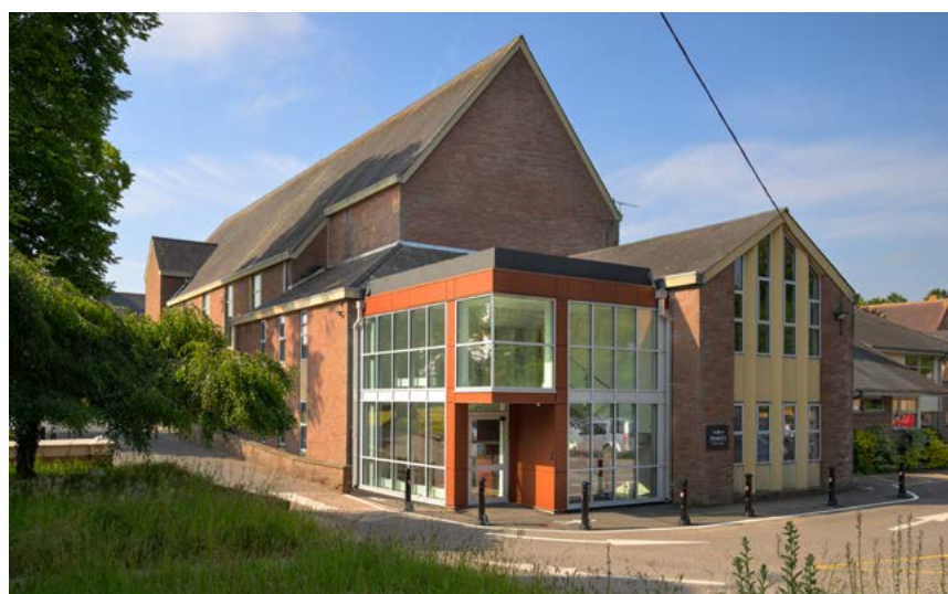
BELOW: Music School extension and modernisation
